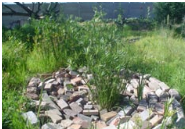
Grey water treatment
